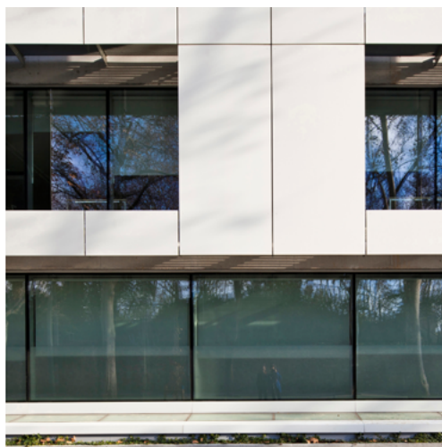
3 在这三座建筑物中，纳瓦罗·巴尔德维格针对每个建筑物的不同立面解决方案和材料的细部/Details of the different façades solutions and materialities in each of the three buildings by Navarro Baldeweg (2.3图片来源/Sources: Eugeni Bach)
